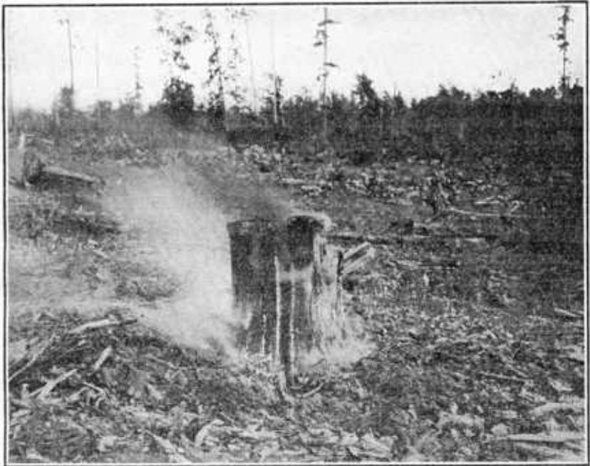
FIG. 4.—Burning a longleaf pine stump as described under Dynamite method. This stump is 22 inches in diameter and was cracked by the use of one-half pound of 40 per cent dynamite. The soil was slightly heavier here than is usually found in longleaf pine land, and it was found unnecessary to dig as deep a trench around the stump in order to induce burning to below plow depth as in places where the soil is sandy.
